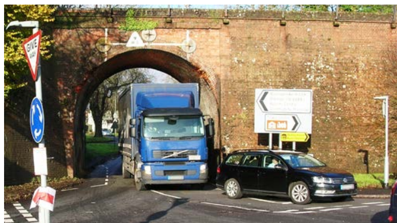
Butts Bridge – a brick arch structure.
