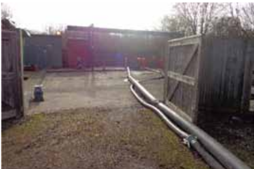
Photo 5 – Additional pumps used to cope with excess flows at Holybourne Pumping Station.
