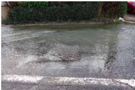
Photo 7 – Surface water ingress into manhole on A32.
