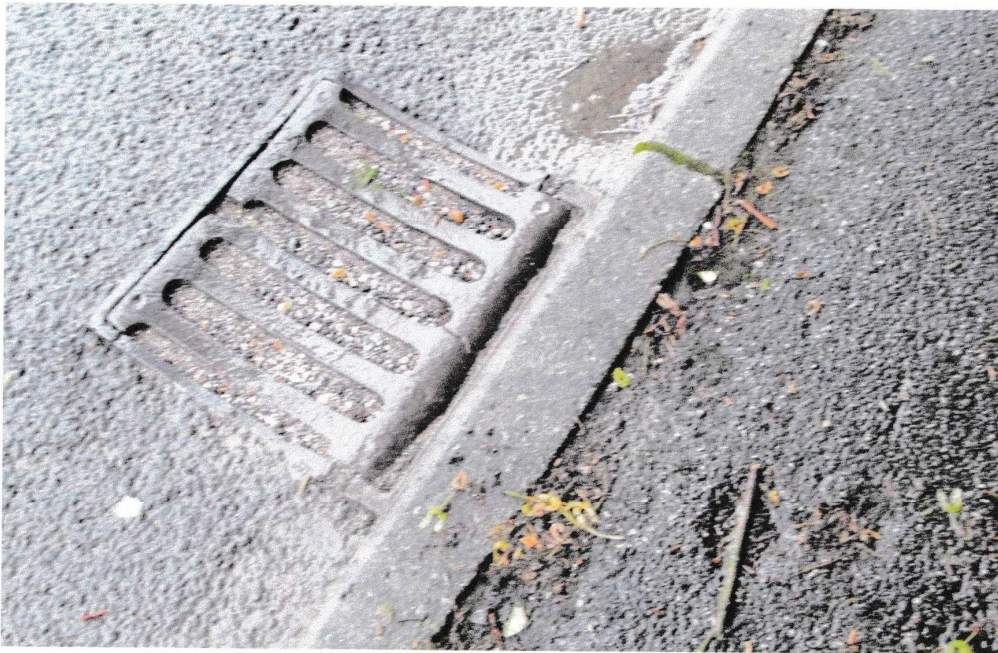
One of many drains monitored since 26/8/2015 that has remained completely blocked.
