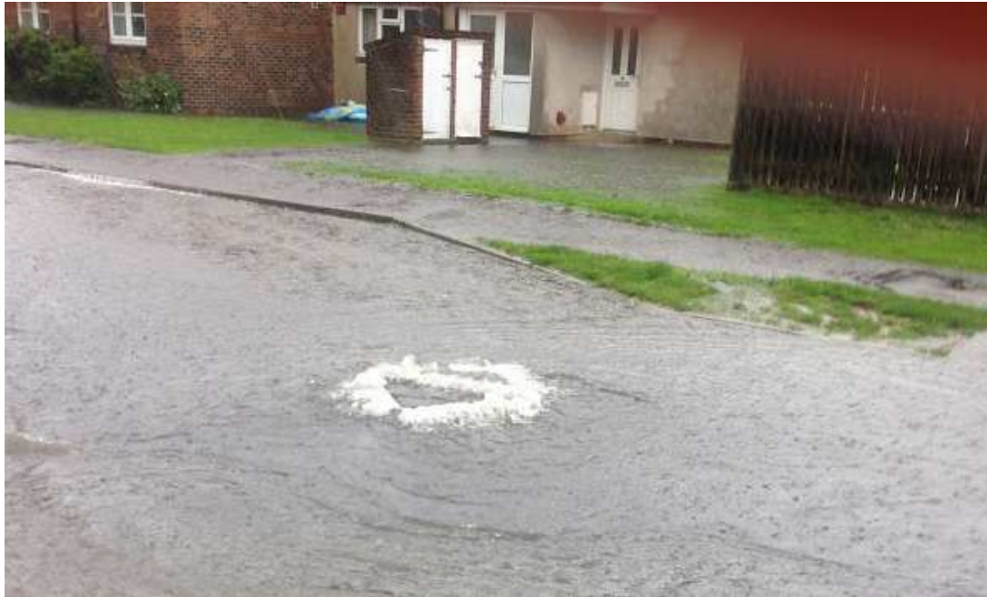
Geales Crescent 26th August 2015- overloaded surface water sewer and overland flow from Spencer Close. The foul sewer also surcharged flooding multiple properties.
